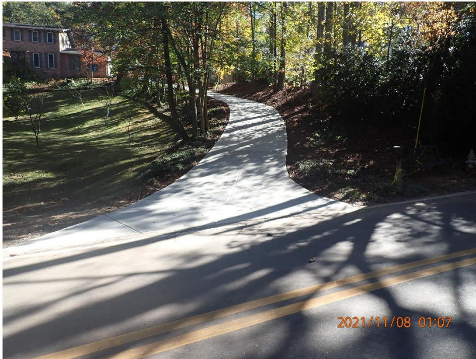
Figure 4 - New driveway at 881 Lakeshore Drive without trench drain
