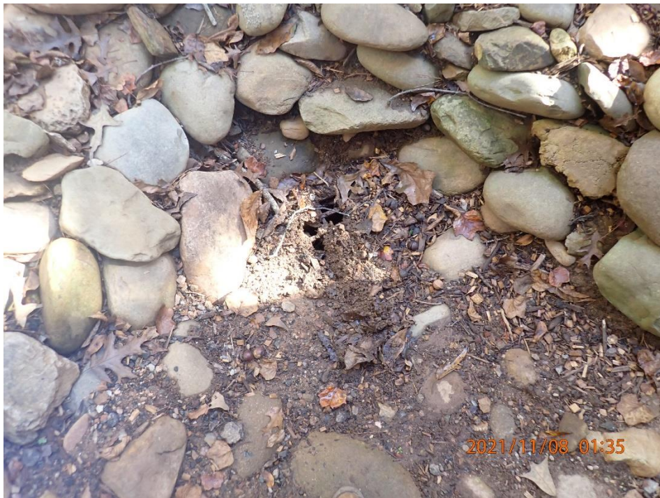
Figure 3 - Structure 158 with clogged grate.
