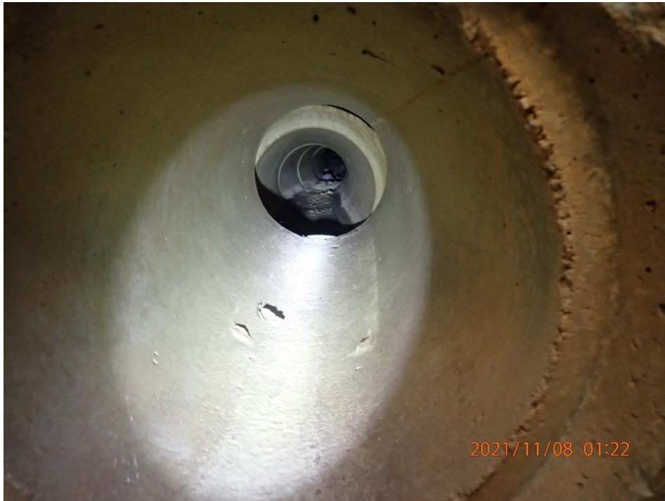
Figure 2 - Pipe under Lakeshore Drive
